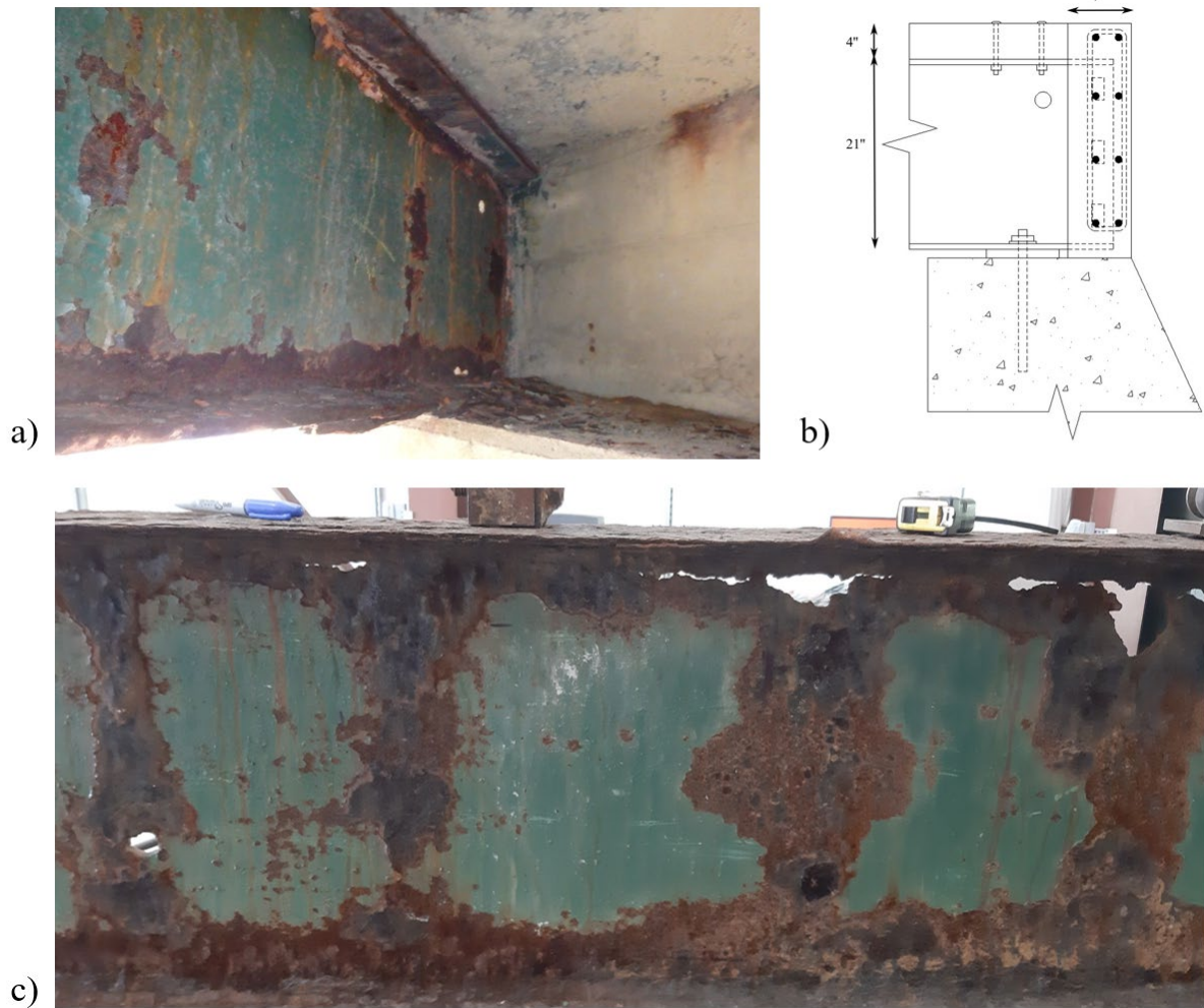
Figure 3.2: (a) In-service configuration, (b) construction details for the support, and (c) web condition at midspan
