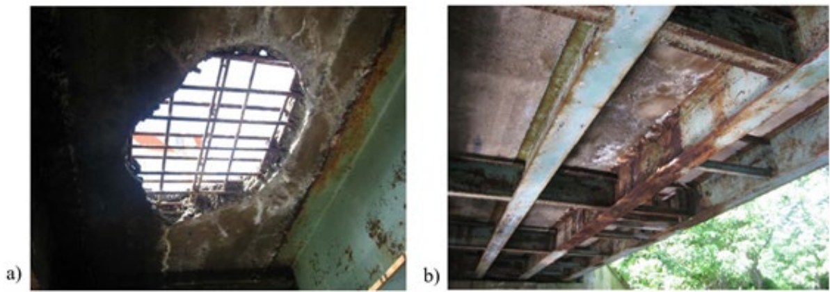
Figure 3.7: a) Hole through the deck, and b) map cracking with heavy efflorescence at the O-03-009 bridge
