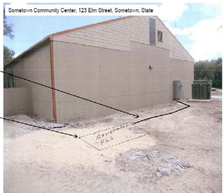
Figure 4. Ground-level photograph showing proposed ground disturbance area.
