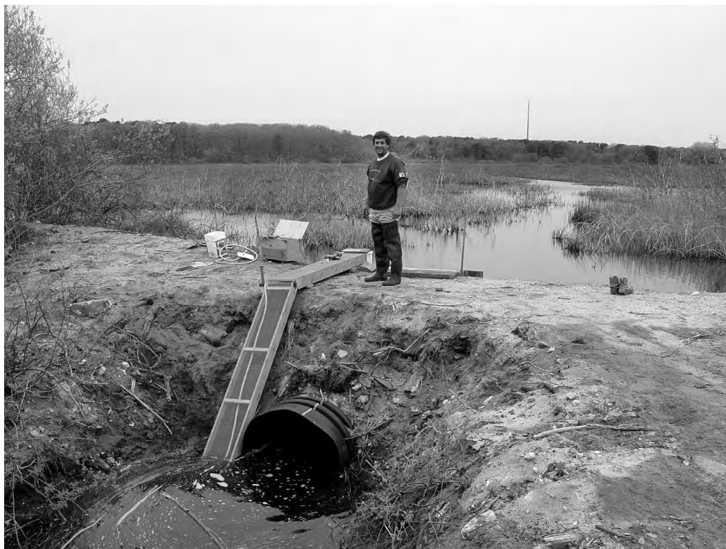
Marine Fisheries' Luis Carmo installing an eel ramp at Cold Brook in Harwich.
