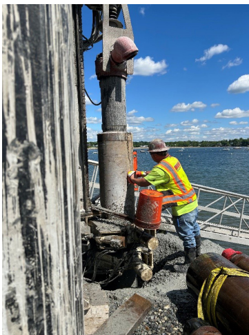
Steel piling being installed this spring for the new Salem Willows fishing pier.
