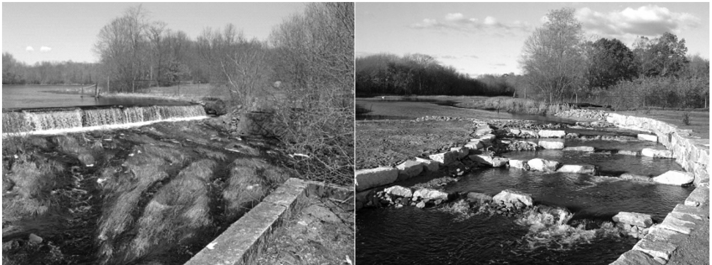
The Acushnet Sawmill Dam prior to (2005; left) and after (2007; right) construction of the stone step pool fishway.
