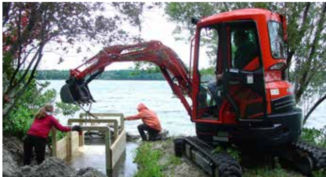
Replacing the wood fishway at Seymour Pond in Harwich.
