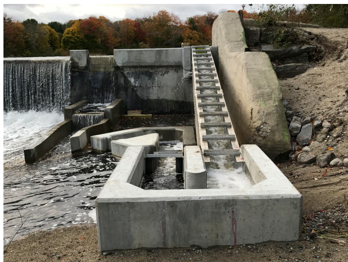
Completed fishway at the Draka Dam.
