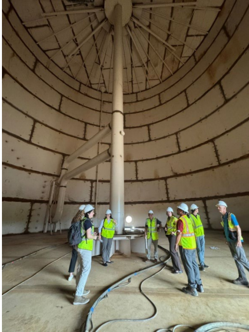
LBE Division Visiting a Thermal Storage Tank at UMass Amherst
