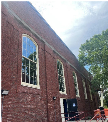
Stoneham Town Hall Window Replacement Project
