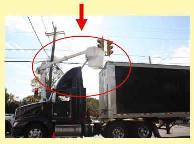
Visual of how each victim was struck by the passing tractor trailer. A truck's bucket and boom should be positioned <u>away</u> from passing traffic, with visible work zone signage.
