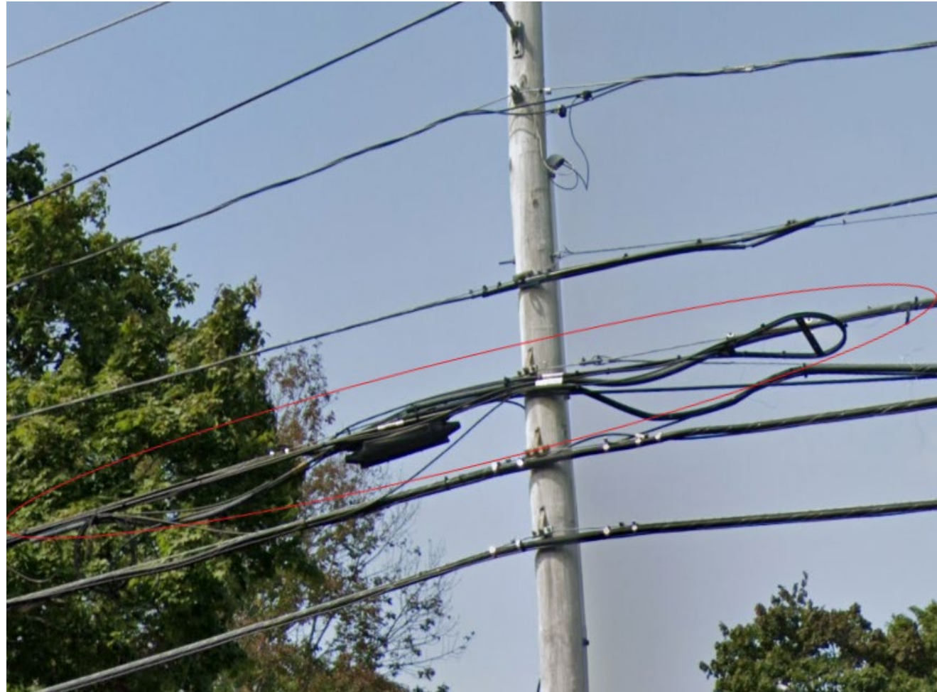
Over-lash detaching from messenger and cable
