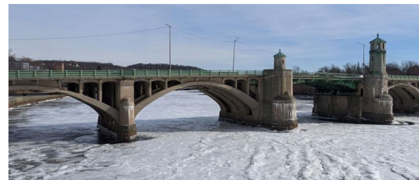
Haverhill – Bridge Replacement, Route 125 over the Merrimack River (Basiliere Bridge)
