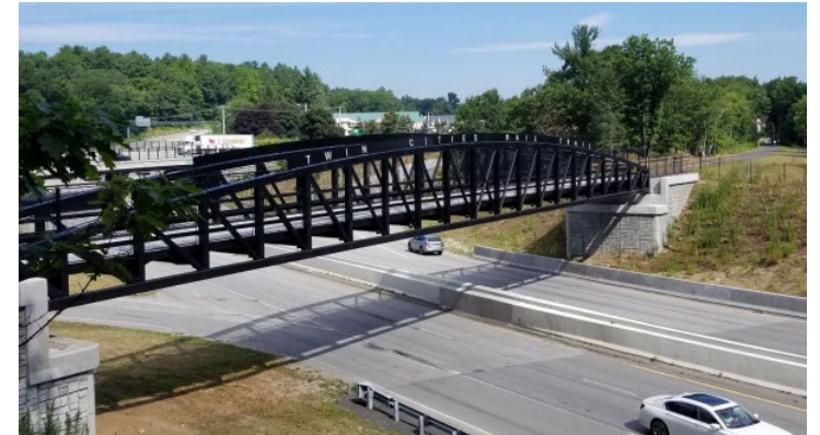
Fitchburg – Twin Cities Rail Trail Construction (Phase II)
