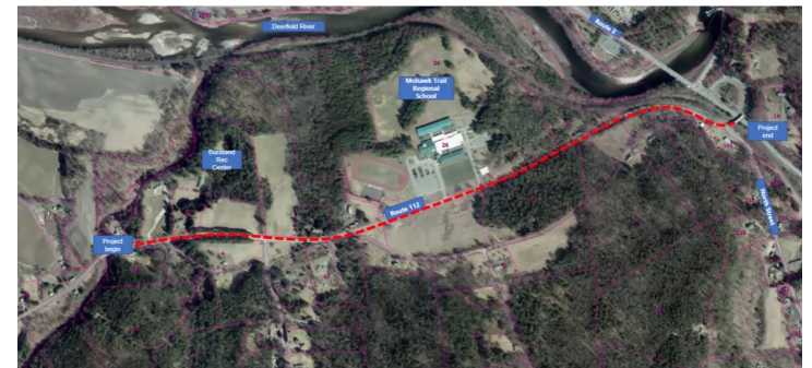
Buckland – Route 112 Project Area
