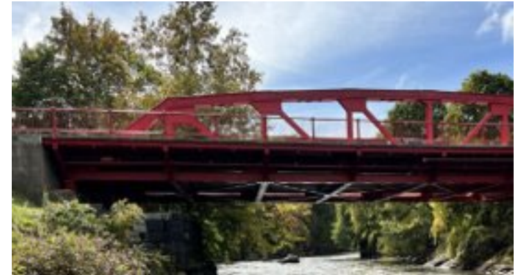
Great Barrington – Brown Bridge over the Housatonic River
