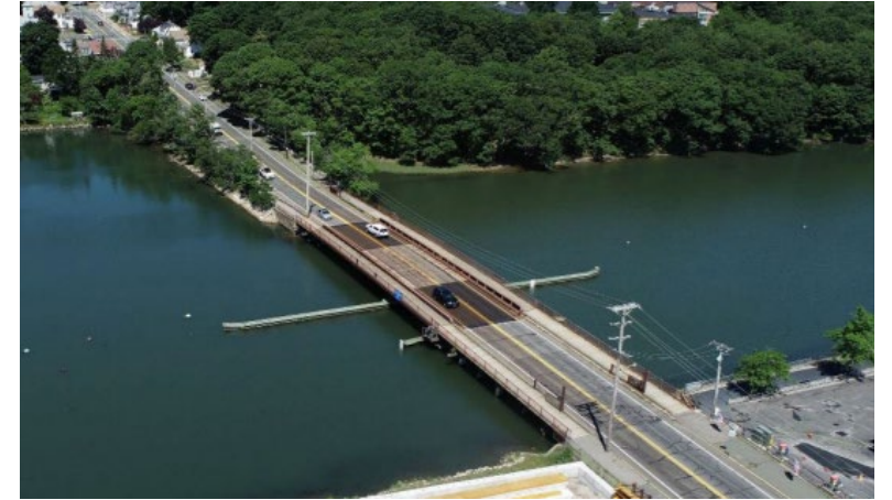
Existing Hall-Whitaker bridge in Beverly
