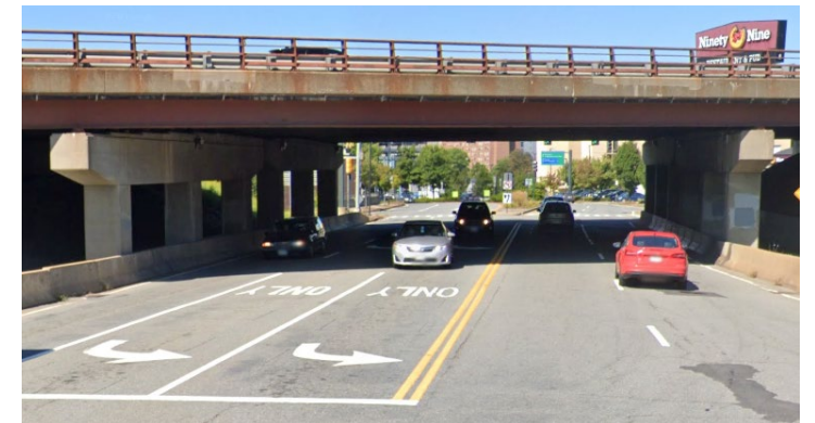
I-290 Bridge over East Central Street in Worcester
