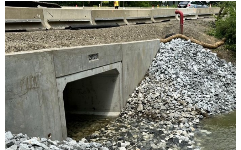
New box culvert on Route 23 in Egremont
