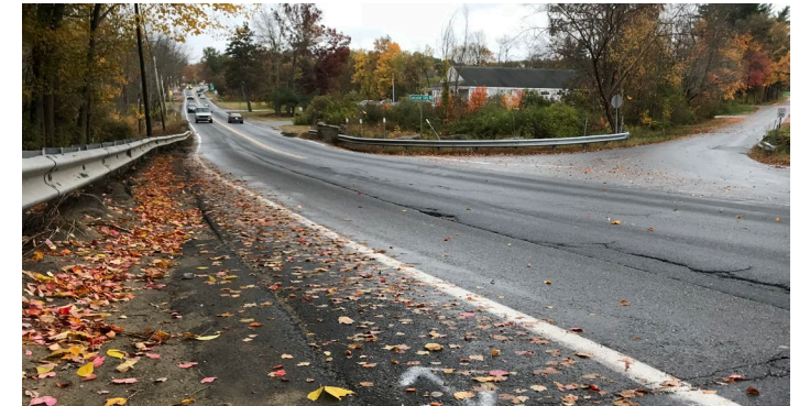
Ayer Road resurfacing in Harvard
