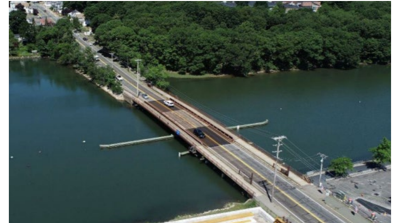
Existing Hall-Whitaker bridge in Beverly
