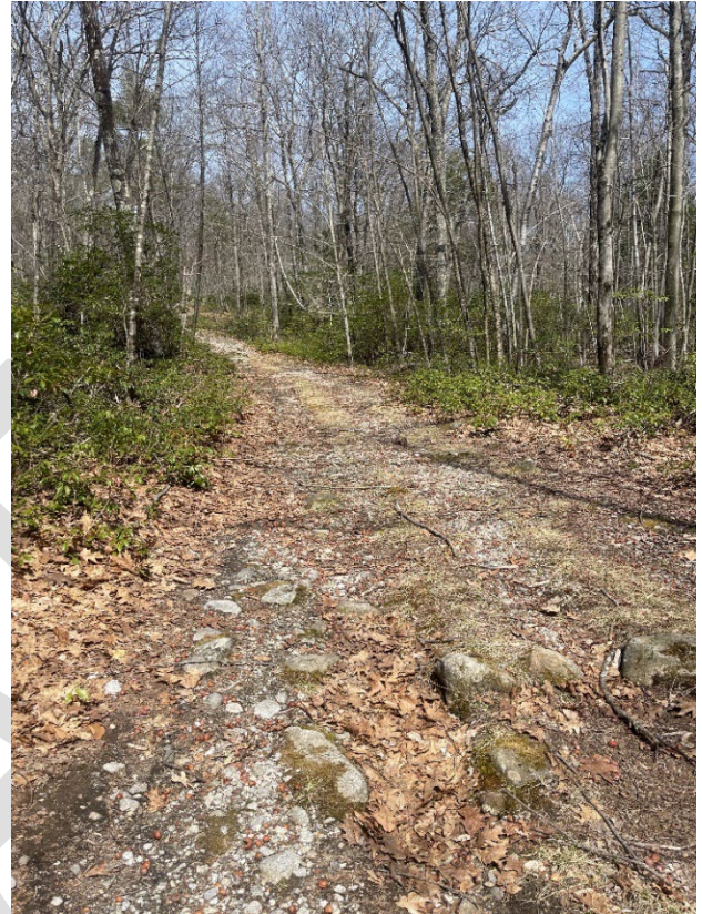
Figure 10. Erosion of Trail Surface
