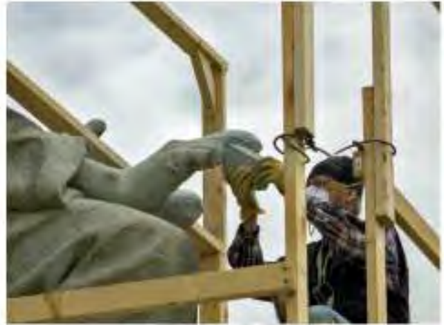
A contractor makes repairs to the missing fingers of the Law figure on Forefathers Monument. (See Appendix K for photo information.)
