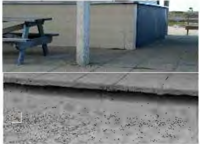
Soil loss from under a concrete walkway near the concession window. At some locations this has already resulted in cracked or collapsed pavement. (See Appendix K for photo information.)
