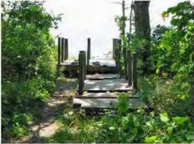
This platform was once connected to stairs to the beach. Erosion undermined the stairs, taking the platform out of use. It now sits in the woods above the beach. (See Appendix K for photo information.)
