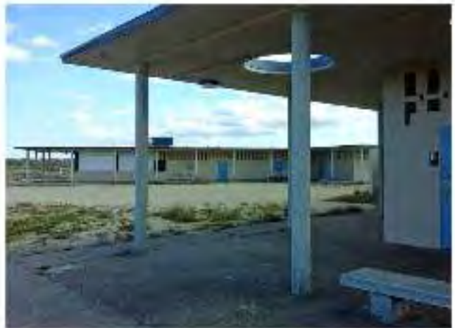
View of Concession/Garage from beach side of Bathhouse. Note the octagonal columns, circular openings in roof, latticework over windows, and concrete bench. (See Appendix K for photo information.)
