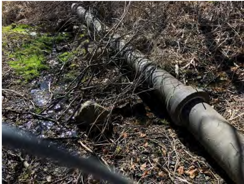
Photo 10 Seeps at Downstream Toe of Left Abutment 4/10/2018
