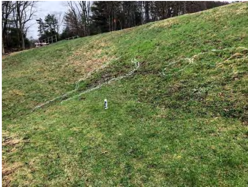
Photo 2 Area of Seeps on Downstream Slope 4/25/2018
