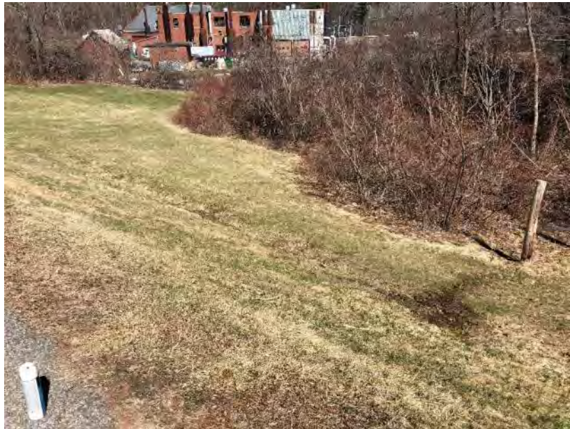
Photo 2 Area of Seeps on Downstream Slope 4/10/2018
