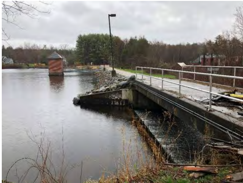
Photo 8 Flashboards Removed, Spillway Invert about El. 31.3 4/25/2018
