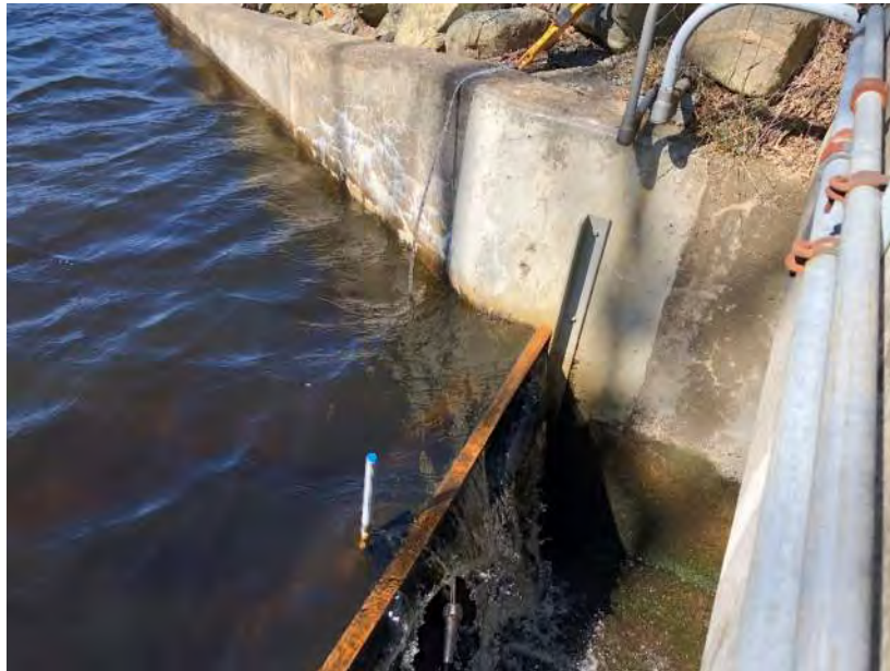
Photo 8 Flashboards at El. 33.3 4/10/2018
