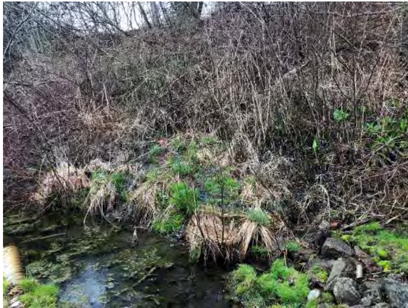
Photo 10 Seeps at Downstream Toe of Left Abutment 4/25/2018
