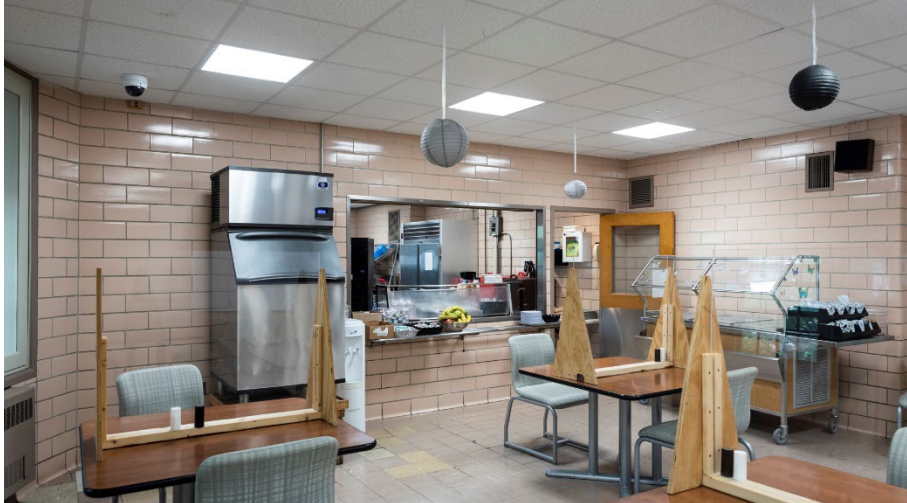
Cafeteria with limited-service kitchen
