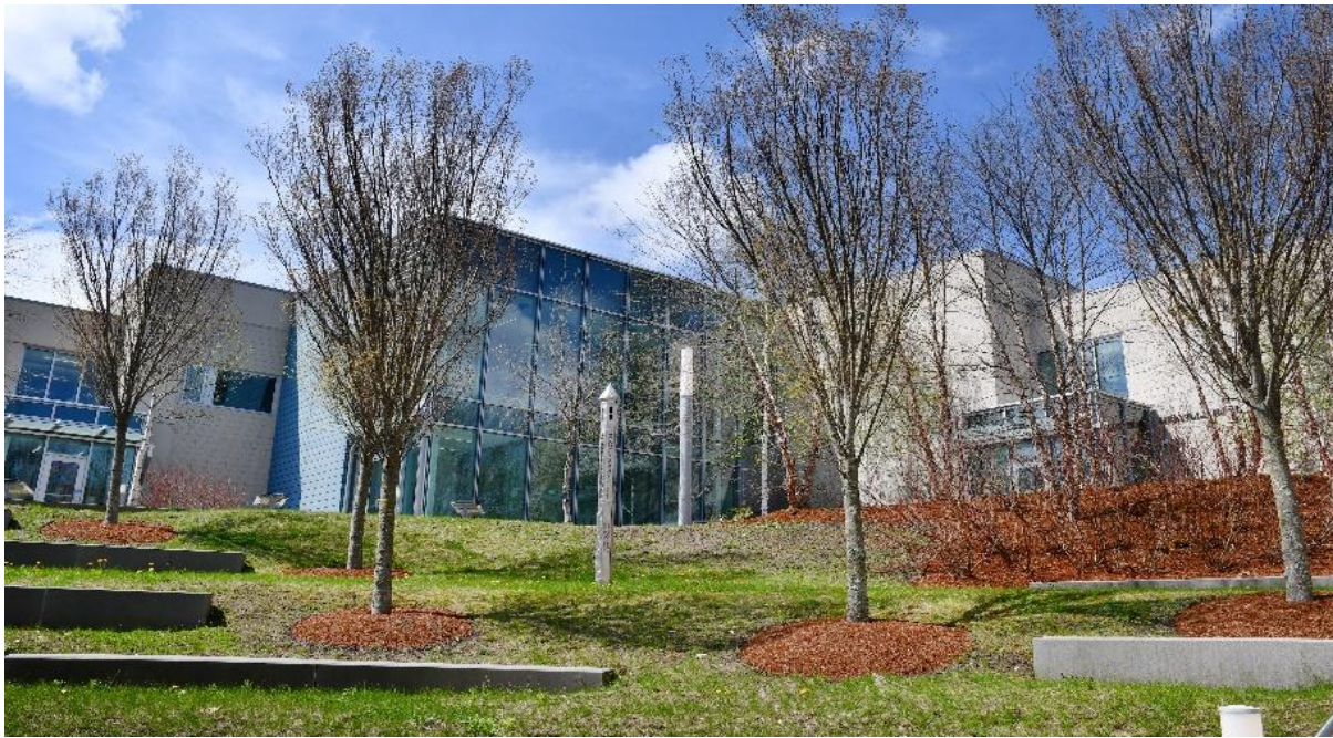
Outside view of Melville Hall, the Connector, and Hawthorne Hall Buildings, Berkshire Community College
