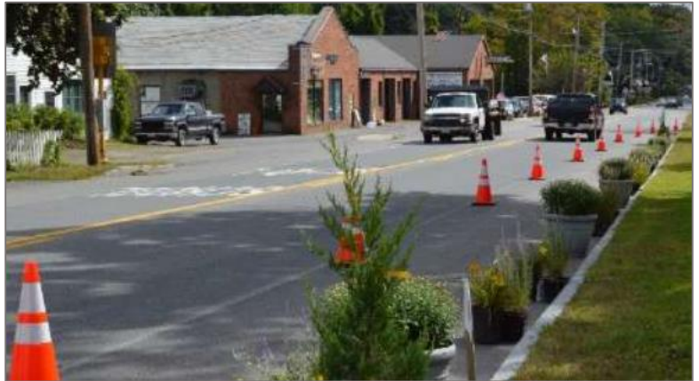
Above: A separated lane for pedestrians and cyclists created using temporary cones and planters.
