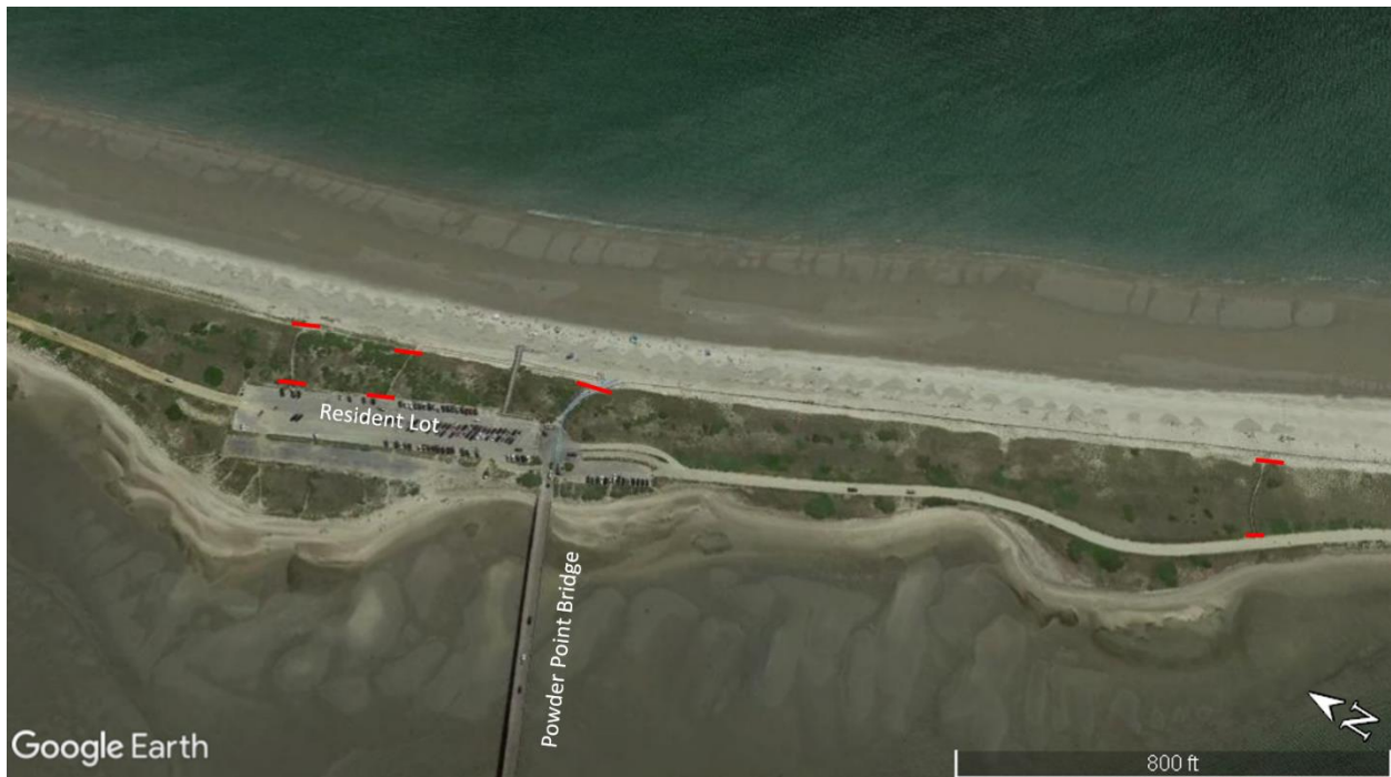
Figure 2. Potential barrier locations in case of two scenarios. The barrier opposite the Powder Point Bridge would be installed if a brood attempts to use that pathway to access the paved parking lot. Barriers at pedestrian pathways will be installed at sunset and removed before the beach opens if Crossover 1 is open to nighttime OSV use and broods exhibit a tendency to cross the road/parking lot to the bayside in this area.
