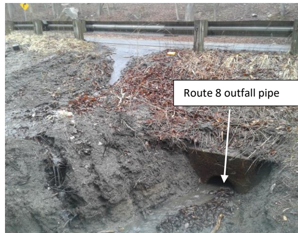
Photo C-8: (above) Curb cut and outfall pipe on Route 8 ROW which leads to an informal stormwater
