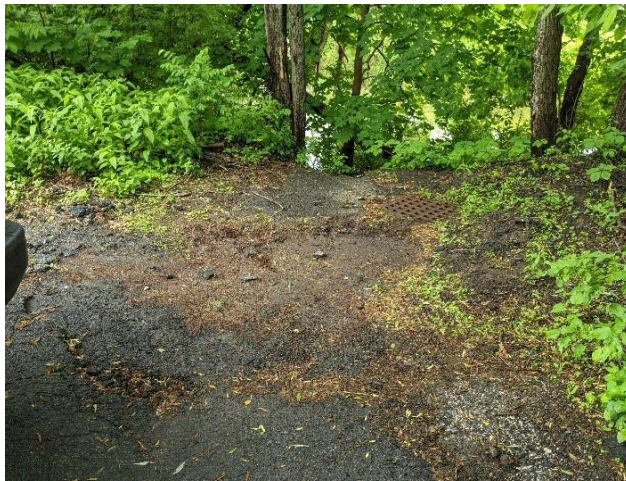
Photo C-1: End of the road runoff avoids the high catch basin and drains to the paved swale left of the basin.
