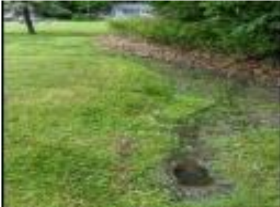
Photo C-5: The outlet of the DPW stormwater pipe is submerged and drains to a yard with no outlet. The outlet should be daylighted and treated with a BMP such as a bioretention basin (Site B).
