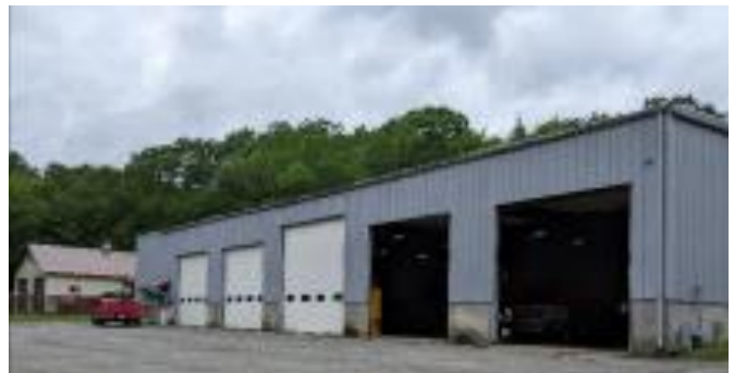
Photo C-4: Front of parking lot and half of the garage are all impervious surface with no stormwater treatment. Infiltration near street may be an option.
