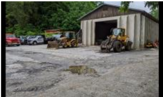
Photo C-3: The main catch basin for the DPW drains half the garage, the lot, and the salt shed. It tends to back up during storms.
