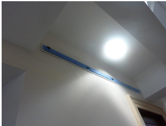
Photo 2 – Linear slot diffuser with filter fabric
