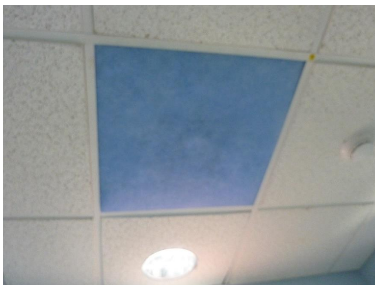
Photo 2 – Linear slot diffuser with filter fabric
