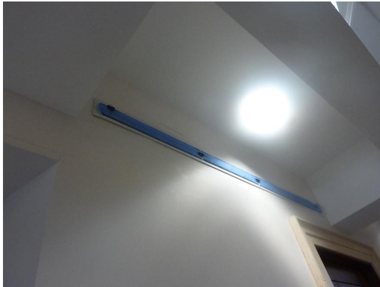
Photo 2 – Linear slot diffuser with filter fabric
