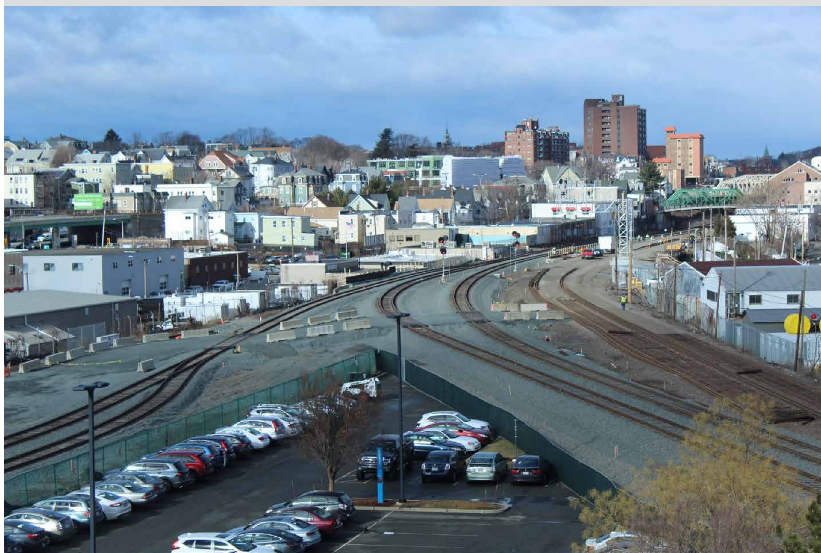
STATION AREA LOOKING NORTHWEST FROM INNER BELT ROAD
