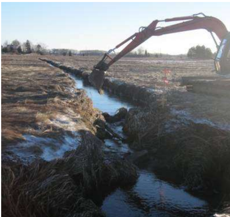
Construction commences to alleviate a >1.5ft impoundment created by gravel debris.
