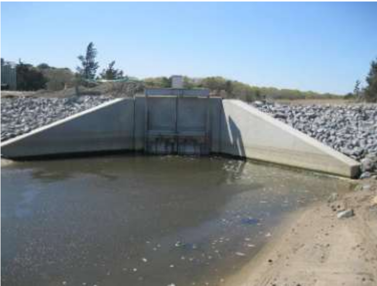
Figure 3: The newly installed box culvert and sluice gate at Stewart’s Creek will restore tidal flow to the 14-acre coastal marsh and wetland.
