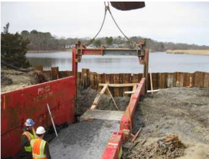
Figure 1: Construction underway at Stewart's Creek – A coffer dam maintains a dry worksite throughout construction. A trench box (red) stabilizes the excavation while the culvert footings are placed.
