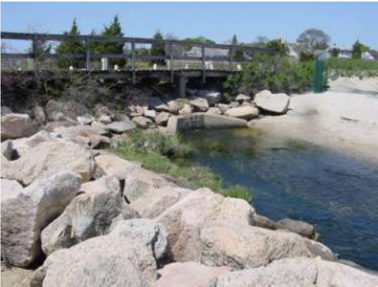
Figure 2: The original three-foot diameter culvert severely restricted tidal flow to Stewart’s Creek, impairing the upstream marsh and reducing nutrient and sediment flushing.
