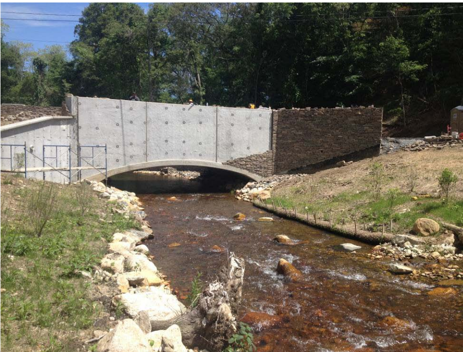
View (looking downstream) of the new Off Billington Street bridge over Town Brook, Plymouth. A rock façade is being applied to the bridge, whose "open bottom" design facilitates the up- and downstream passage of fish and wildlife.
