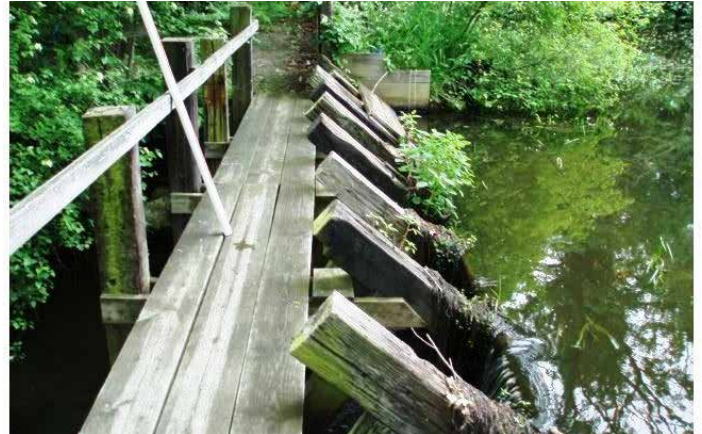
Barstowe's Pond Dam left spillway
