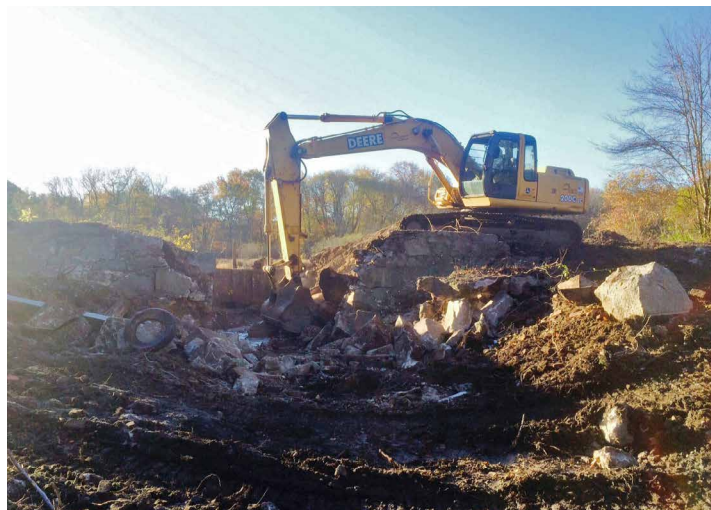
Above: Rattlesnake Brook Dam Below: The removal of the Rattlesnake Dam in process.
