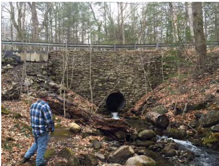
Ashfield DPW Director, Tom Poissant looks at the undersized, perched culvert slated for replacement.
