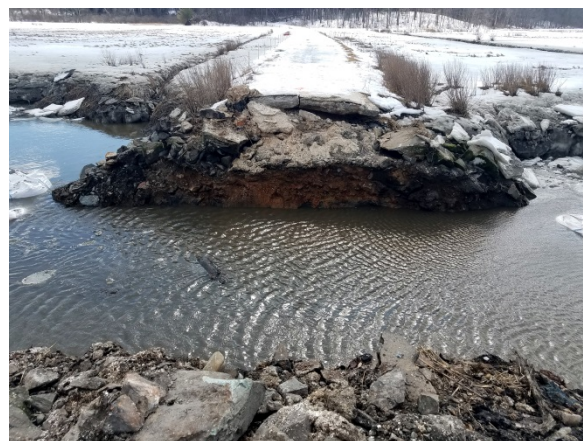
Restoration work underway at Kent's Island in Newbury
