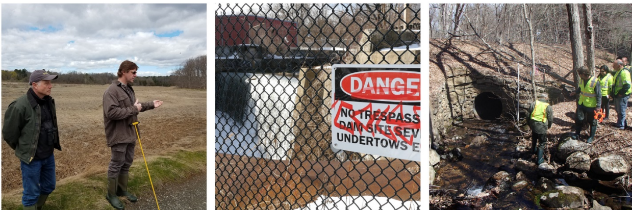
Left: Site visit as part of the Great Marsh Restoration project. Middle: View of the Tel-Electric Dam. Right: Culvert Replacement Training being held at the Rice Corner Culvert in Brookfield
