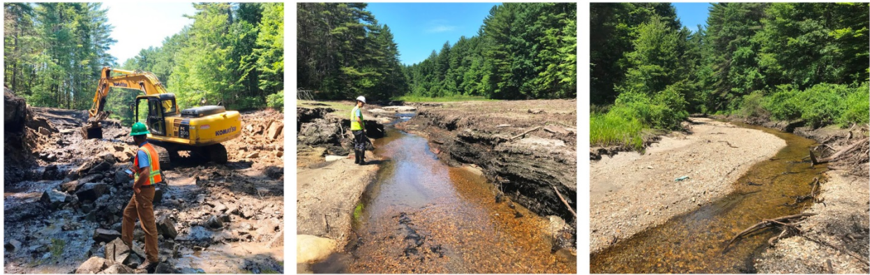
Left to Right: Dam removal well underway; channel forming about midway through previous impoundment; channel forming through the upper section of former impoundment.
