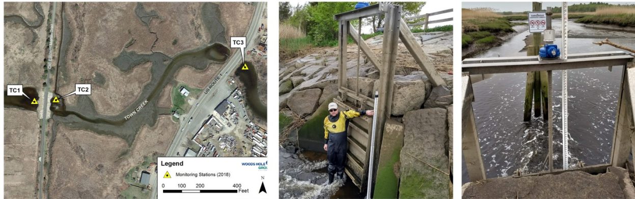
Left: Location of tidal monitoring equipment at Town Creek. Middle and Right: Measuring opening size and elevation at the Town Creek Tide Gate (Figure and photos by Woods Hole Group, Inc.).
