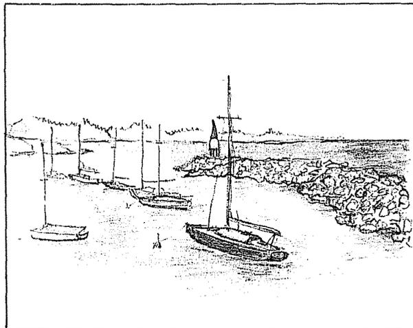
Jetties are linear barriers built of large rock or concrete. They are positioned to reduce the effects of storm wave surge or the force of strong currents. Jetties may be built parallel to offshore bays and river mouths to protect boat harbors or perpendicular to the shore to protect navigation channels of harbors and marinas.
