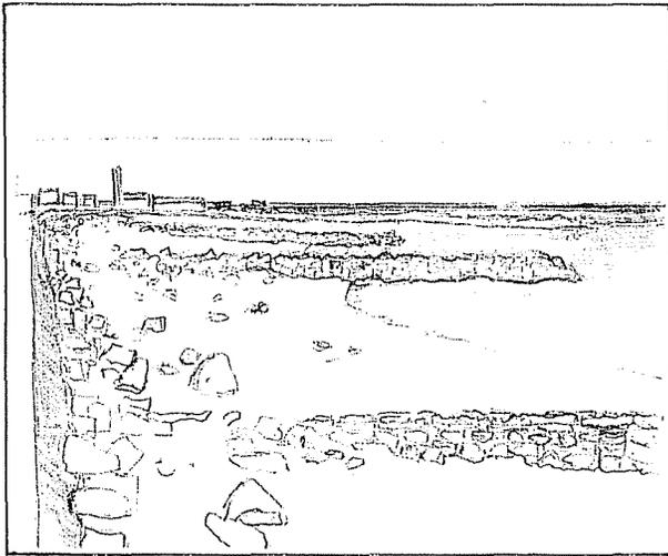
Groins are linear structures built perpendicular to the shore. Their purpose is to interrupt the normal pattern of littoral drift and wave refraction to prevent local shoreline erosion or encourage sand deposition. They are built of large rocks or concrete and their length and height vary with the strength of littoral flow, tide levels and storm strength.
