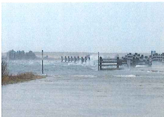
Figure 5: Flooding and overtopping of the Dike Bridge on Chappaquiddick Island during the March 2018 Nor'easters
