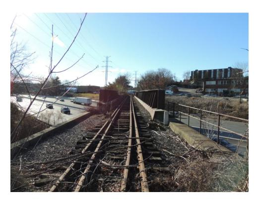
Over MBTA Fitchburg Line, Weston: 1896 Riveted Lattice Thru Truss on Stone Abutments
