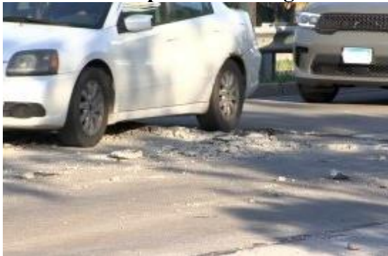
Roadway buckling on DuSable Lakeshore Drive during a heat wave on June 21, 2022 Source: NBC Chicago
