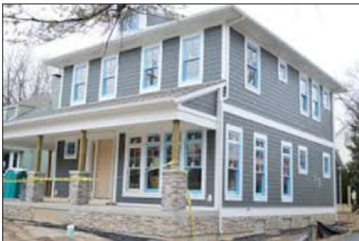
Figure 1: Front and east side of the building
