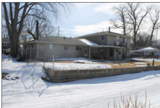
Figure 4: View looking east toward properties across the channel
