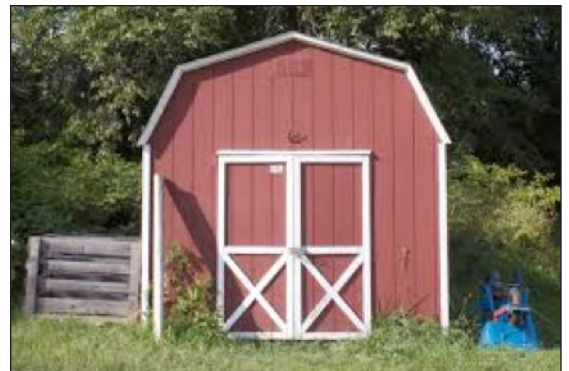
Figure 6: Outbuilding constructed in 1975 is located 55 feet west of the back of the house. This structure will be removed as part of the demolition project.
