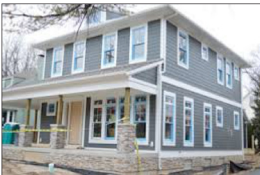
Figure 1: Front and east side of the building
