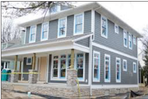
Figure 1: Front and east side of the building
