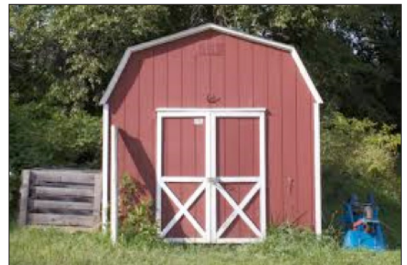
Figure 6: Outbuilding constructed in 1975 is located 55 feet west of the back of the house. This structure will be removed as part of the mitigation project.
