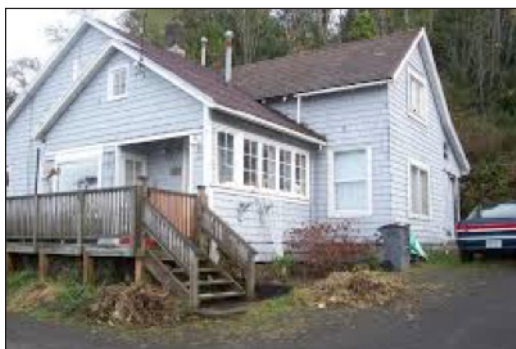
Figure 4: Back and west side of the house
