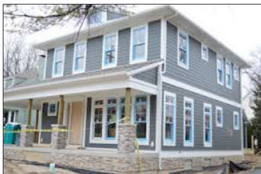
Figure 3: Front and east side of the building
