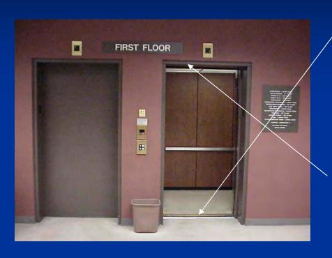
**Door Gibs** - Devices at the bottom of horizontal sliding door panels, which stick into sill grooves and eliminate door panels swinging in or out.
