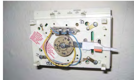
Figure 4.1: Existing Mercury Non-programmable thermostat in the Old Edgell Library
