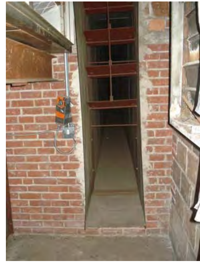
Figure 18.1: Existing return air damper in HV-1 Mixed Air plenum
