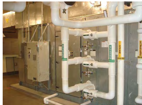
Figure 5.1: Existing Air Handling Unit serving Cameron Middle School
