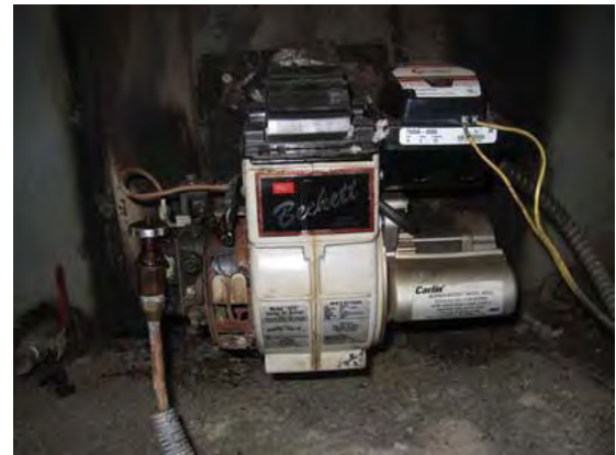
Figure 9.1: Existing oil burner installed in the Old Edgell Library
