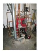
Heating for the building is provided by a single H.B. Smith, cast iron sectional hot water boiler. This boiler uses # 2 heating oil and has an output capacity of 174.8 MBH. Heating hot water is distributed via two fractional horsepower zone pumps to baseboard radiation located throughout the facility.
