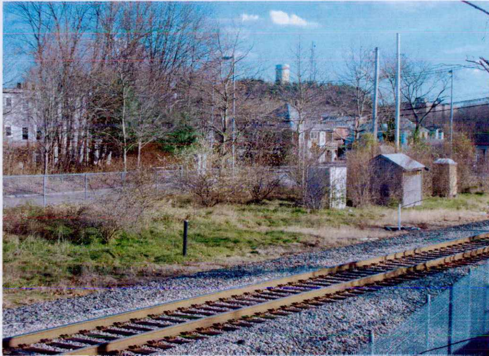
GEC Project No. 1424-2350. November 26, 2012. 106 Hale St. Bridgewater, MA. Monitoring wells and sheds for LNAPL recovery system.
