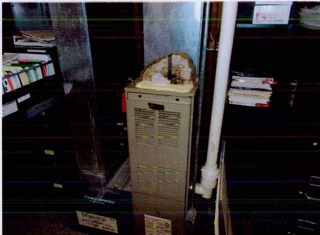
GEC Project No. 1424-2350. November 26, 2012. 106 Hale St. Bridgewater, MA. Gas fired heating unit.
