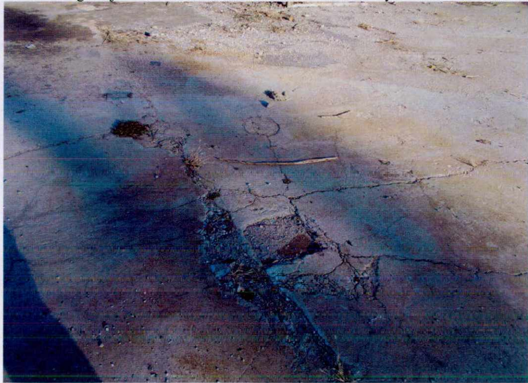
GEC Project No. 1424-2350. November 26, 2012. 106 Hale St. Bridgewater, MA. Former building foundation with likely column footings.
