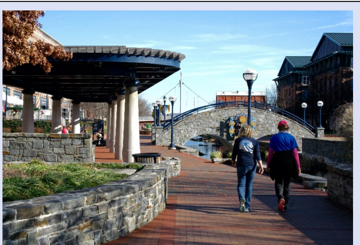
Exhibit 9. Frederick, Maryland. While Carroll Creek Park began as a flood control project, its evolution as a cultural and recreational amenity has helped stimulate economic development. More than $150 million in private investment is underway along the park.
