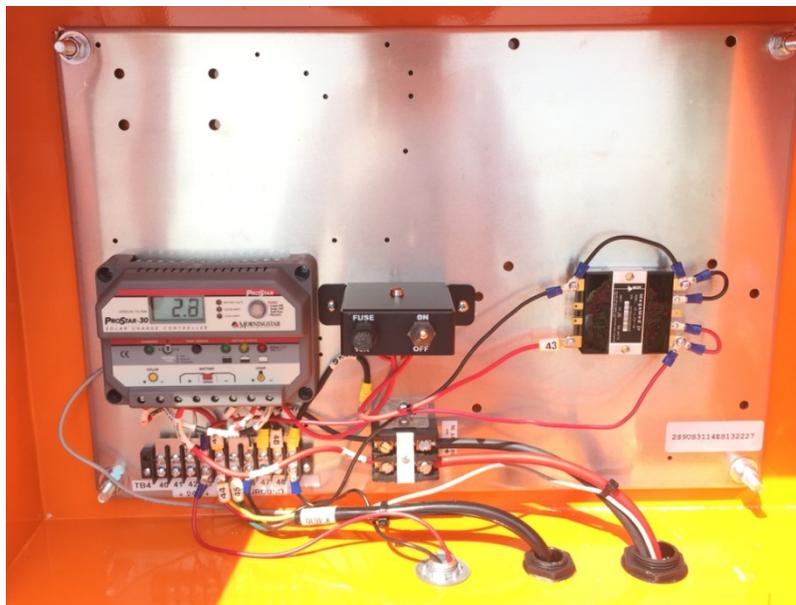
**Figure 3.11: Solar controller box**
