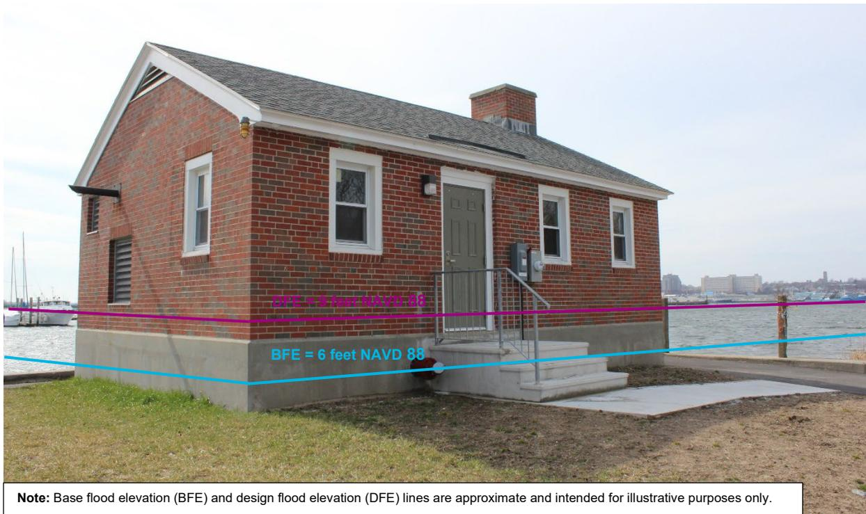
**Note:** Base flood elevation (BFE) and design flood elevation (DFE) lines are approximate and intended for illustrative purposes only.
