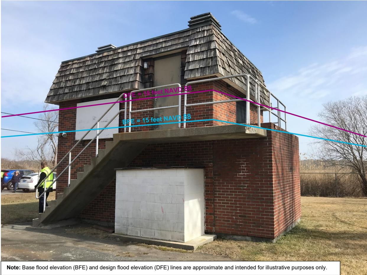
**Note:** Base flood elevation (BFE) and design flood elevation (DFE) lines are approximate and intended for illustrative purposes only.
