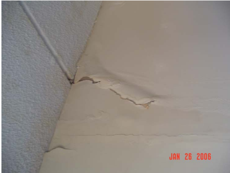
667-4 Elderly Development Bates and Tower, 57 Bates Street, #502 Kitchen – Wall and Ceiling Have Water Damage from Leak in Roof
