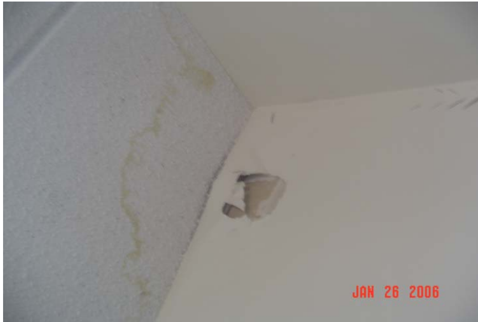
667-4 Elderly Development Bates and Tower, 57 Bates Street, #502 Living Room – Wall Has Water Damage from Leak Near Bay Window
