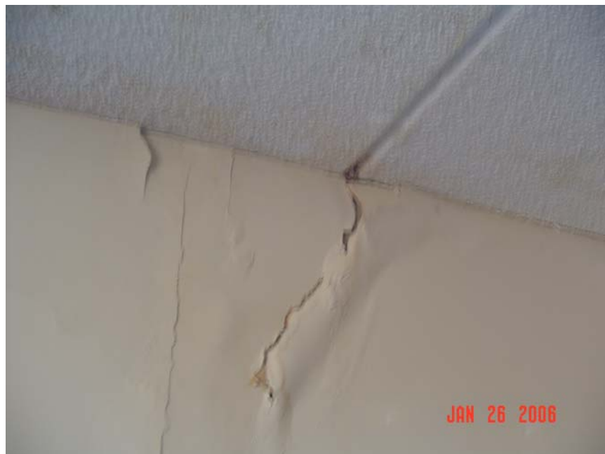
667-4 Elderly Development Bates and Tower, 57 Bates Street, #502 Kitchen – Wall and Ceiling Have Water Damage from Leak in Roof
