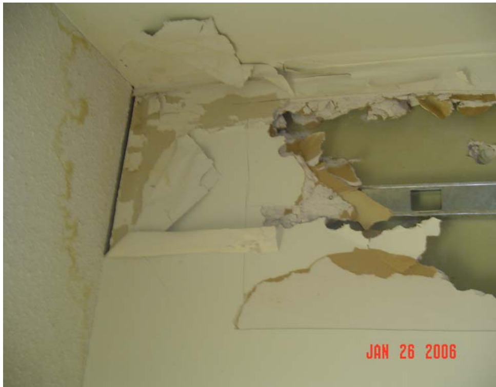
667-4 Elderly Development Bates and Tower, 57 Bates Street, #502 Living Room – Wall Has Water Damage from Leak Near Bay Window
