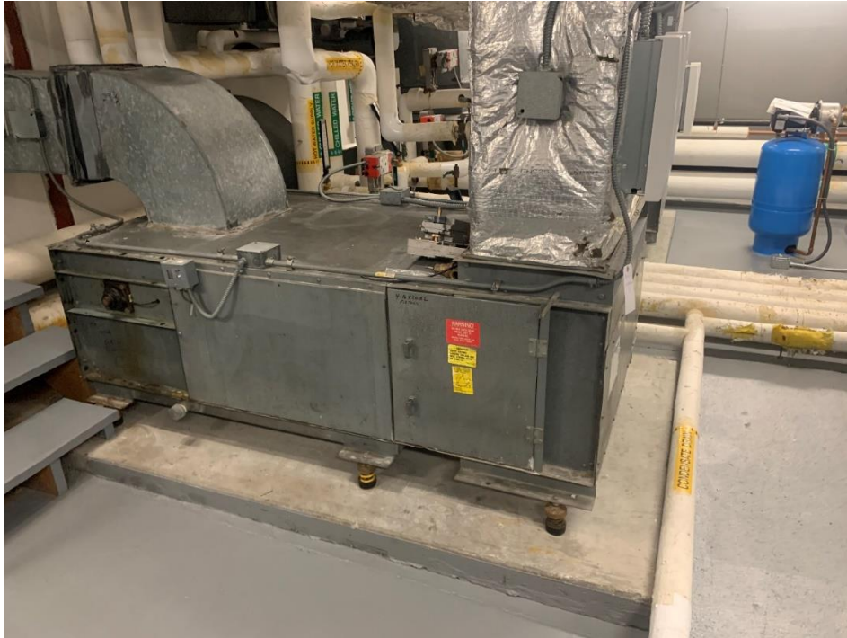
Photo 1 – Typical Courtroom Air Handler
