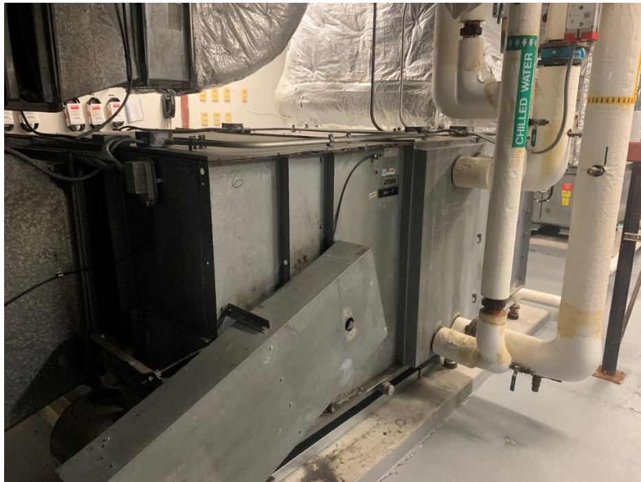
Photo 2 – Typical 100% Outdoor Air Handling Unit
