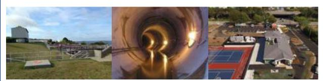
The upgraded Primary Treatment Facility and Sodium Hypochlorite Storage Facility at the WWTF (left). The CSO tunnel, bored through solid rock, toward the end of its construction (center). The recently completed President Avenue CSO screening and disinfection facility at Veterans Memorial Bicentennial Park (right).
