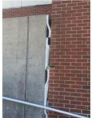
Settlement exhibited in building joint and stairs at Pump House No. 2. Settlement has resulted in piping and electrical service failures.
