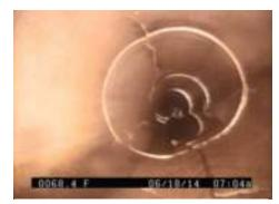
Closed-circuit television image showing a cracked pipe
