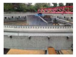
*Clarifier No. 3 is out of service. The center drive cage sheared and requires replacement.*
