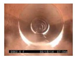
Closed-circuit television image showing offset joints
