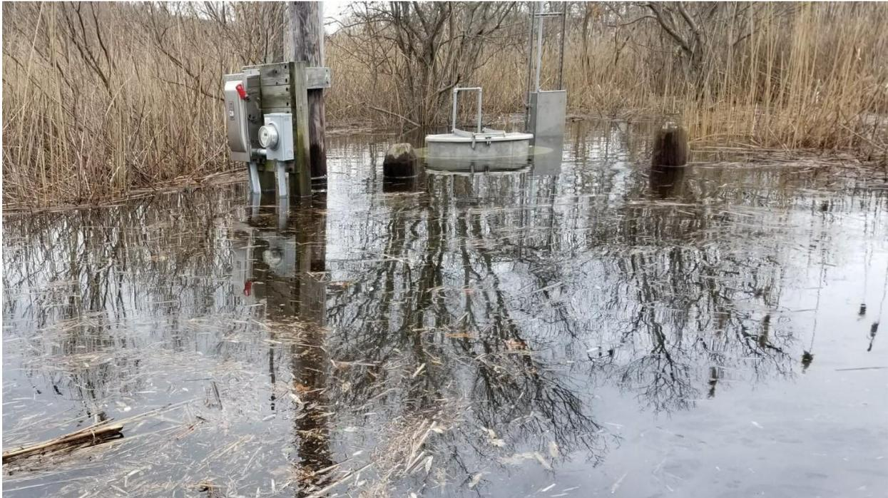
Figure 1: Park Road Lift Station During a Flooding Event in 2018.
