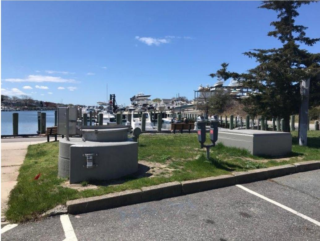
Figure 3: Inner Harbor Lift Station Located at the Head of Falmouth Inner Harbor
