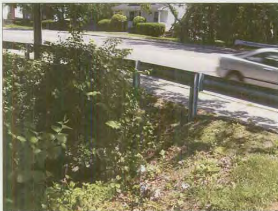
Photo 5: Area Adjacent to First Downstream Crossing
