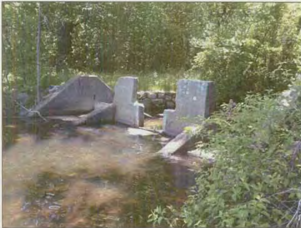
Photo 3: Upstream Face and Spillway
